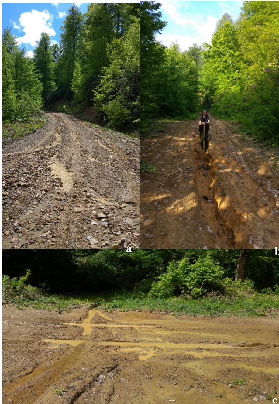
Figure 3. Unpaved road segment samples. a Sediment transport along the rills that form on the road segment. b Highly eroded road surface. c Erosion on the node where two road segments intersect
