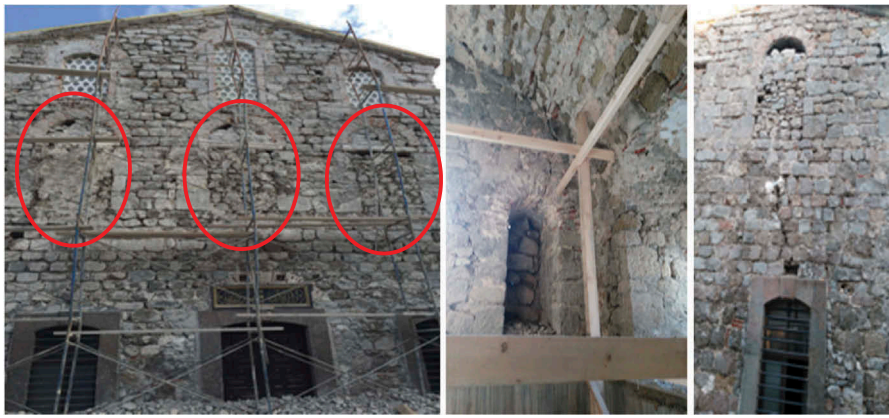
Figure 5. Views of closed window openings on the exterior walls.
