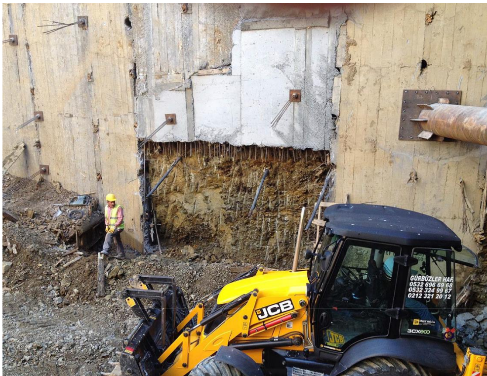
Figure 8: Top-down construction of wall and encountered in-situ soil anchors
