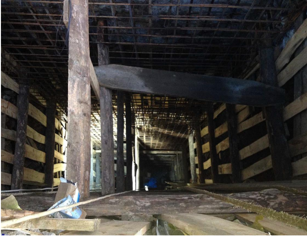
Figure 5: Reinforcement installation for the wall
