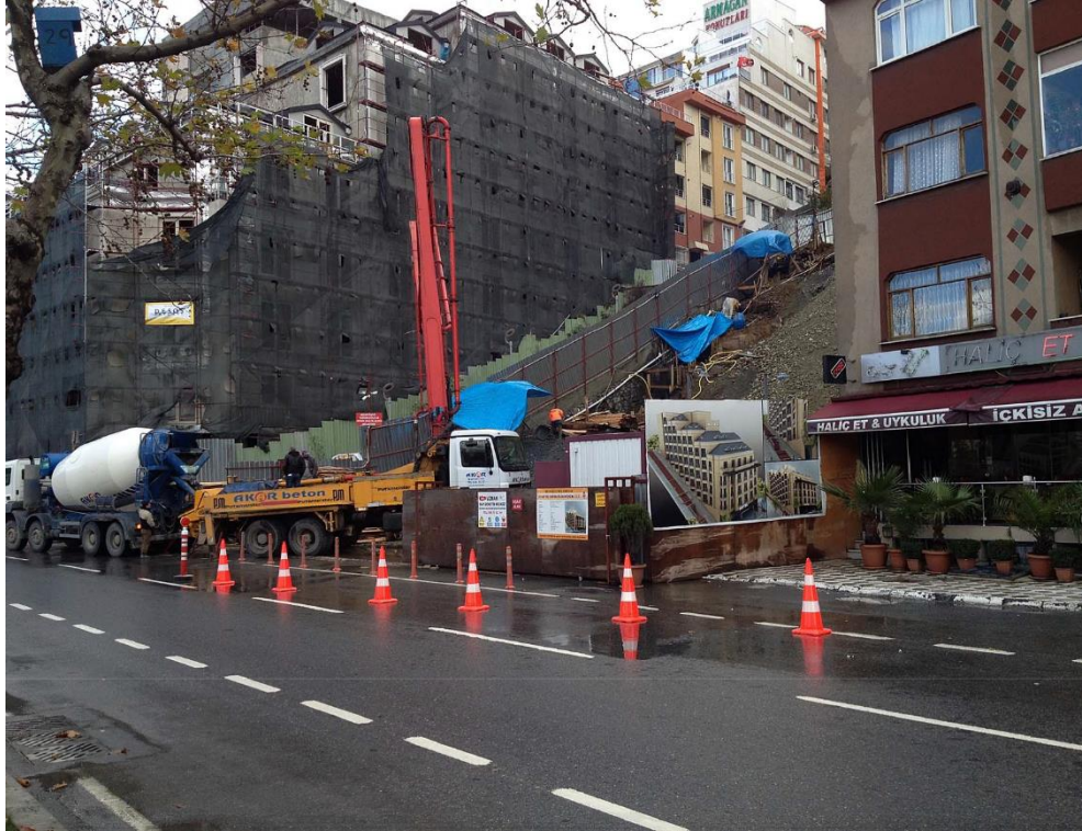
Figure 3: Early stage of construction at second lot
