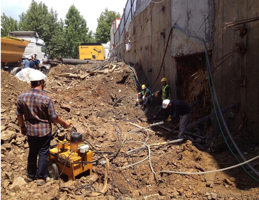
Figure 7: Stressing the soil anchor from the second lot as tendon
