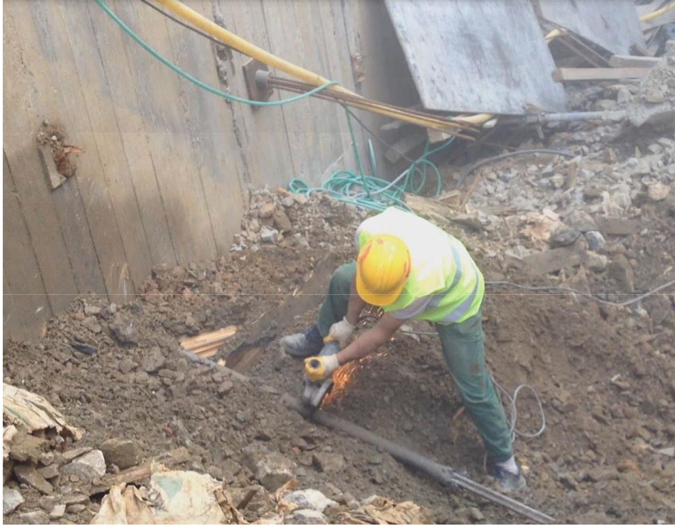
Figure 9: Cutting the soil anchor to the required length to be used as tendon
